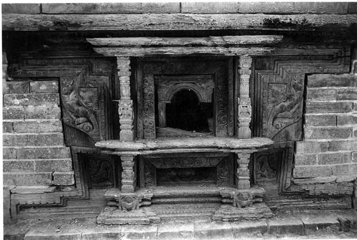
Existing Condition of Decorative Carved Window ( Gh jhyah ) PHOTO OF GH JHYAH AT WEST FACADE
