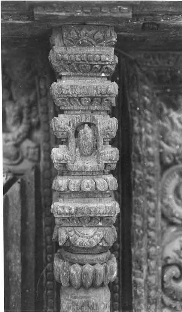
Left: extended timber column on main entrance doorway. Face of the small deity is worn due to weathering
