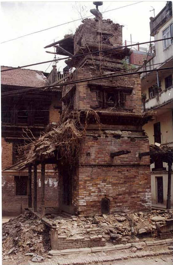
South facade: September 1997
