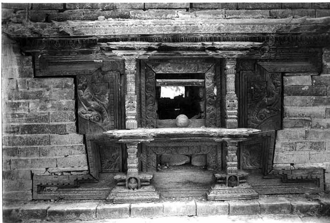
Existing Condition of Decorative Carved Window ( Gh jhyah ) PHOTO OF GH JHYAH AT NORTH FACADE
