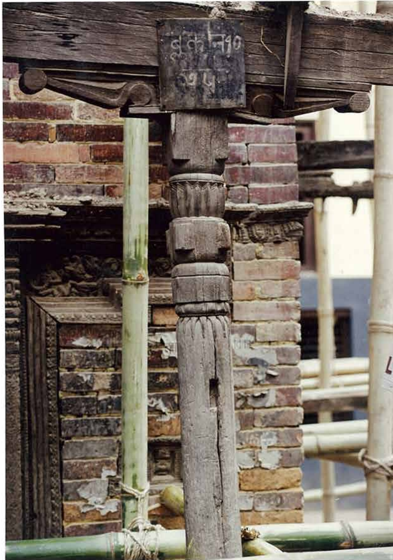
Original column and capital assembly, west elevation, fall, 1998. The notch accepts lost roof strut.
