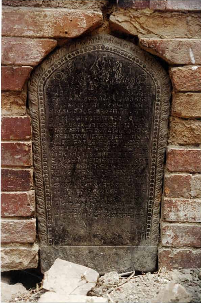
Stone inscription on ground floor level on south facade
